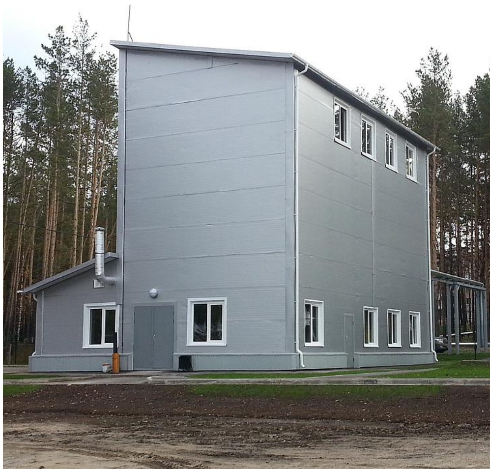
Local WWTP of the boarding house «Lesnaya Dacha». Capacity 500 m 3 per day. 2012, Tomsk region, Russia
