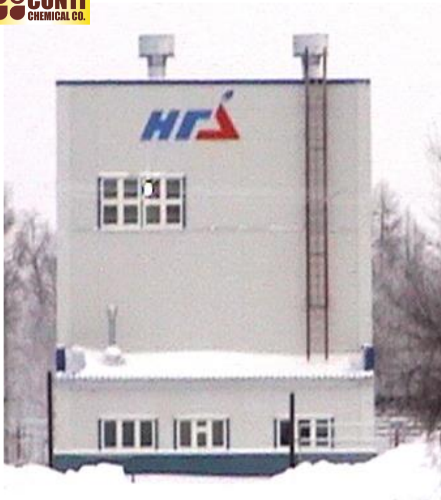
Local WWTP of Vyngapur natural gas field, «Gazprom» branch. Capacity 150 m 3 per day. 2006, Yamalo-Nenetsk region, Russia
