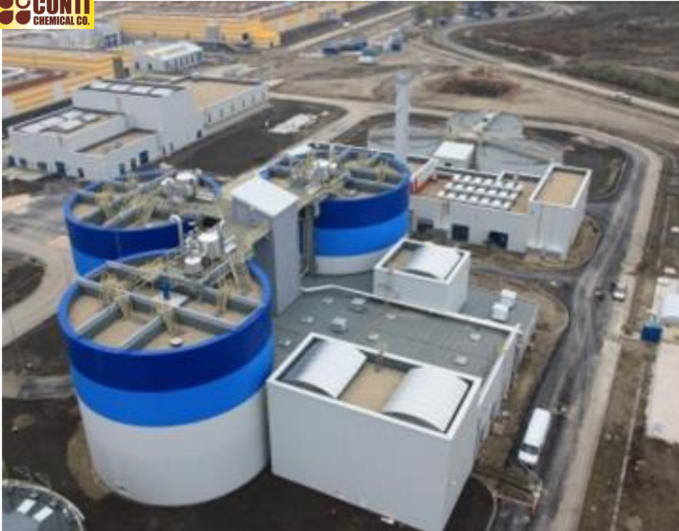
Sludge treatment at the Southern WWTTP of Budapest (front-end technical solution). 2016-2017, Hungary
